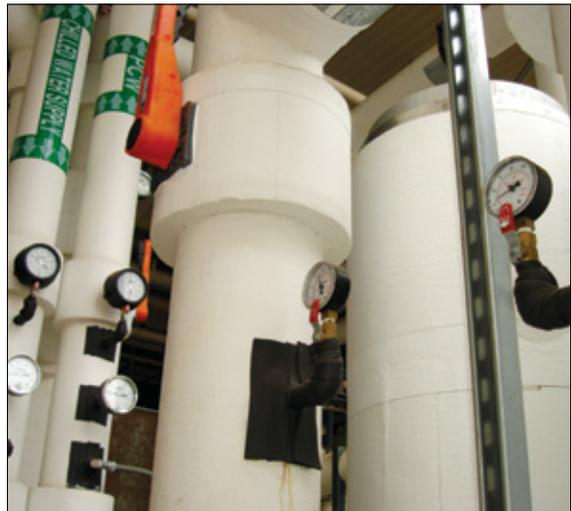
New Process Cooling Water system for MDL cleanrooms with increased capacity and control for instrument cooling needs.
